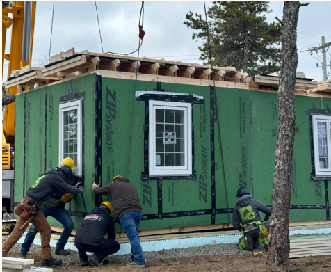
Truro resident Jody Mellander's ADU unit during construction in winter 2023-24.
